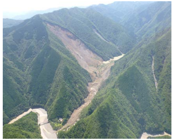
Landslide dam at Akadani Area, Gojo City, Nara Pref.
