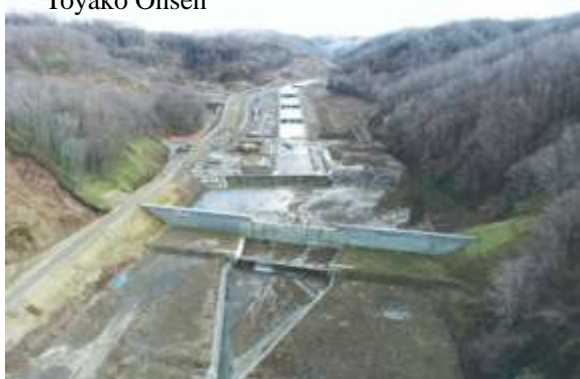
Sediment control facilities after earthquake (Hidakahoronai River)
