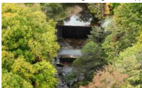
Heiwa Sabo dam in Kotoni-Hassamu
