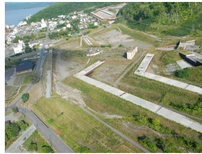
Nishiyama River Sabo dam at Mt. Usu
