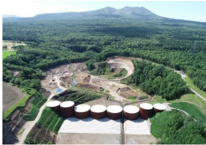
Oboppu River Sabo dam at Mt. Tarumae
