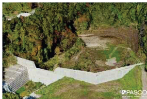
3D models of SABO dams are developed and used to create an integrated 3D SABO GIS map and to support facility management.
